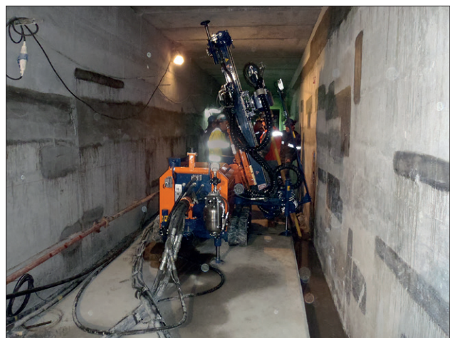
Drilling in confined galleries
