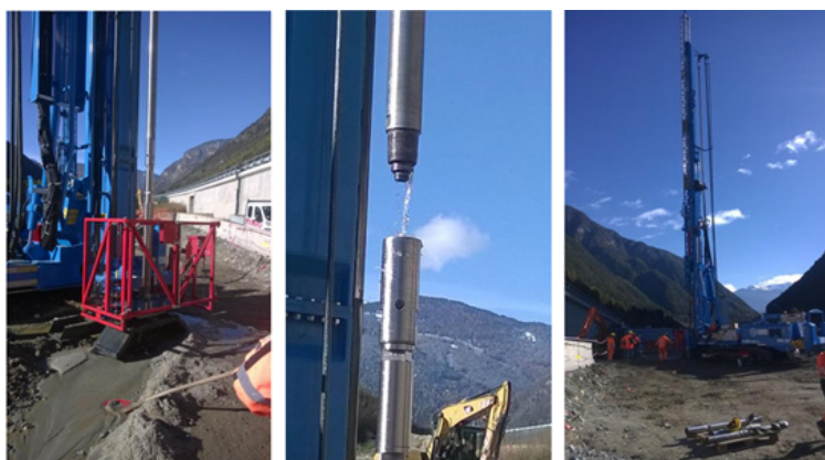
Left: W120 Hammer and monitor, Middle: Monitor and triple fluid rods, Right: Solimec SM 28 in action
