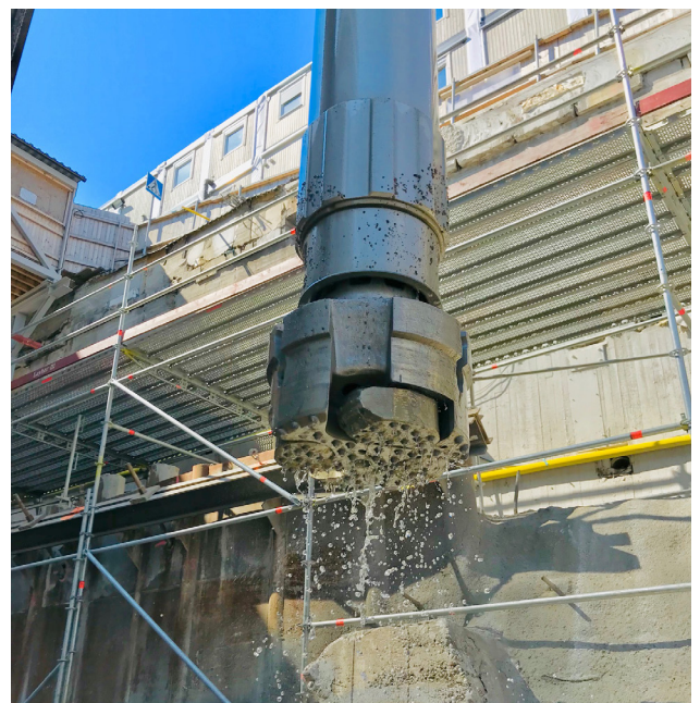
W280 in action at Slussen, Stockholm, Sweden
